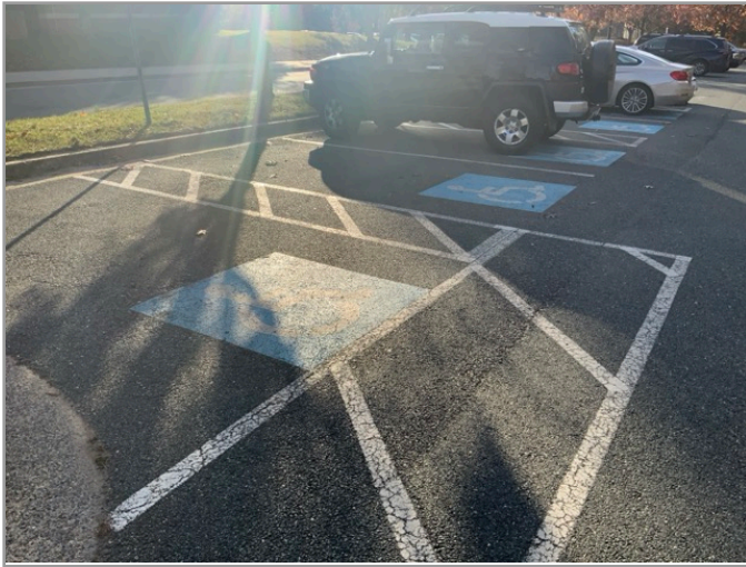
OVERVIEW OF ACCESSIBLE PARKING AREA
