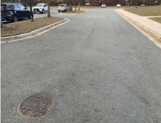
31 - ASPHALT PARKING LOTS
