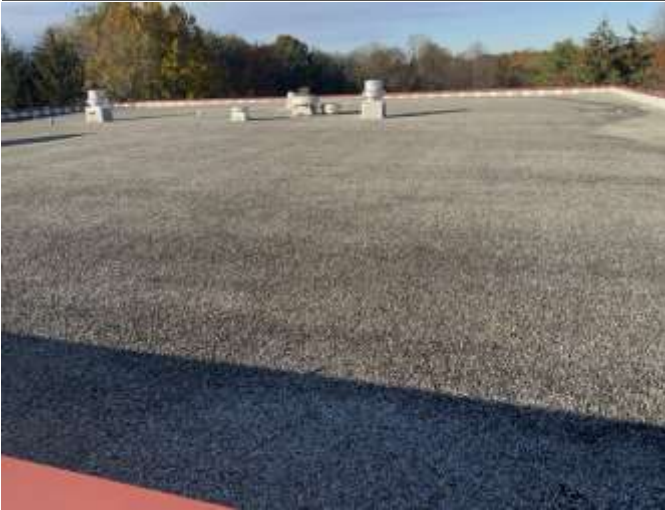
7 - BUILT UP ROOFING
